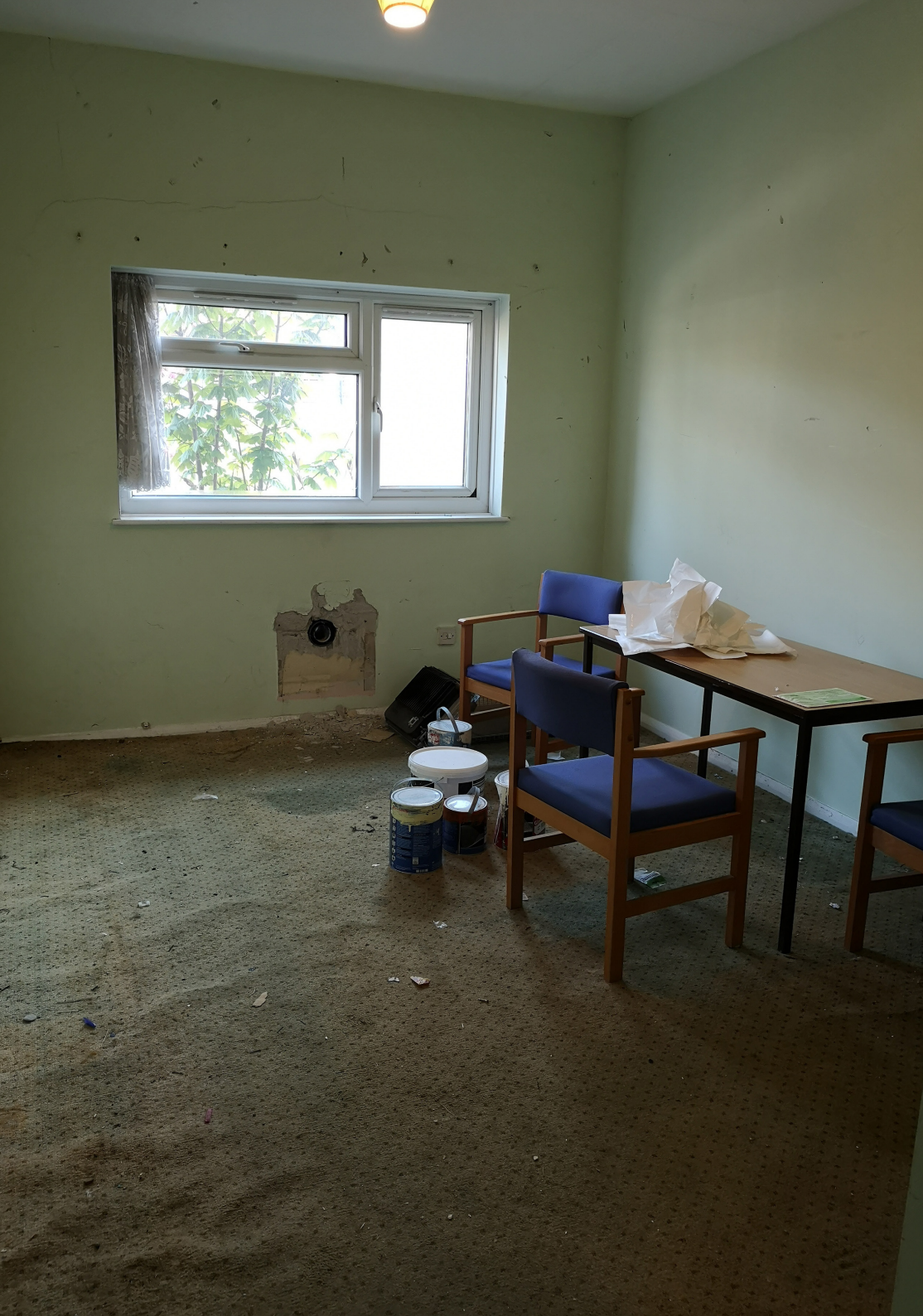
Visitors' Room renovation
